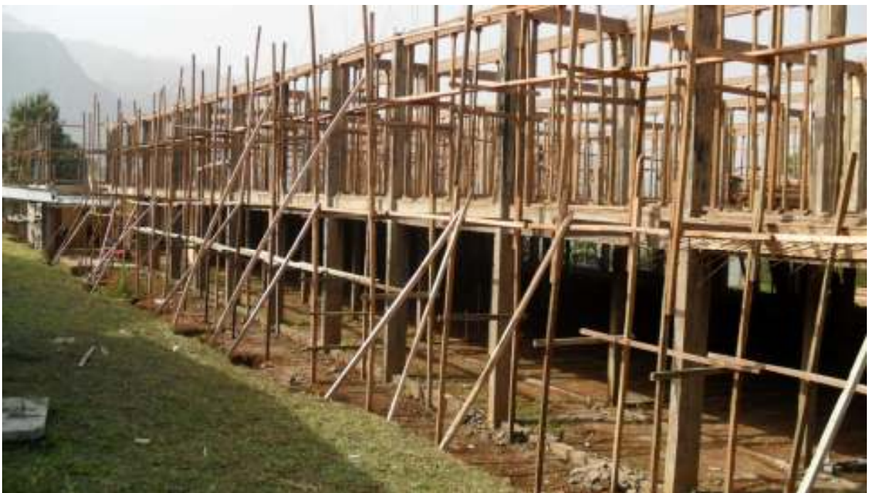
MBH NEW OPD UNDER CONSTRUCTION – FRONT VIEW
