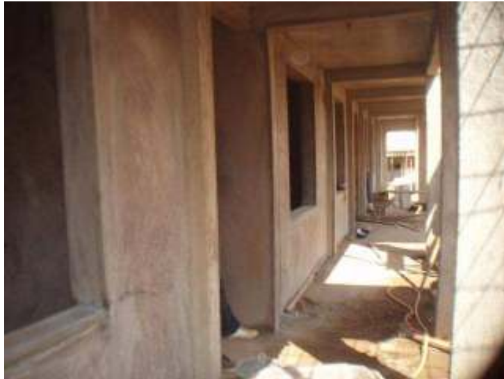
Ground Floor of New BBH Eye Department Being Completed
