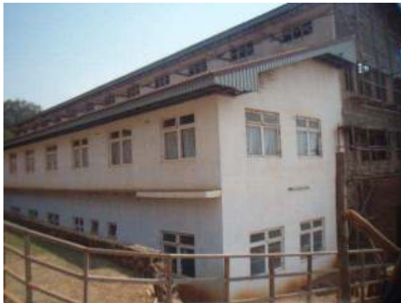
BBH OPD COMPLETED SIDE VIEW
