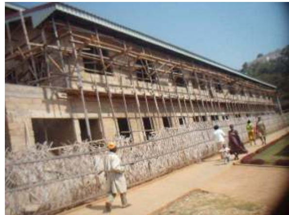
BBH OPD SIDE VIEW – PENDING COMPLETION
