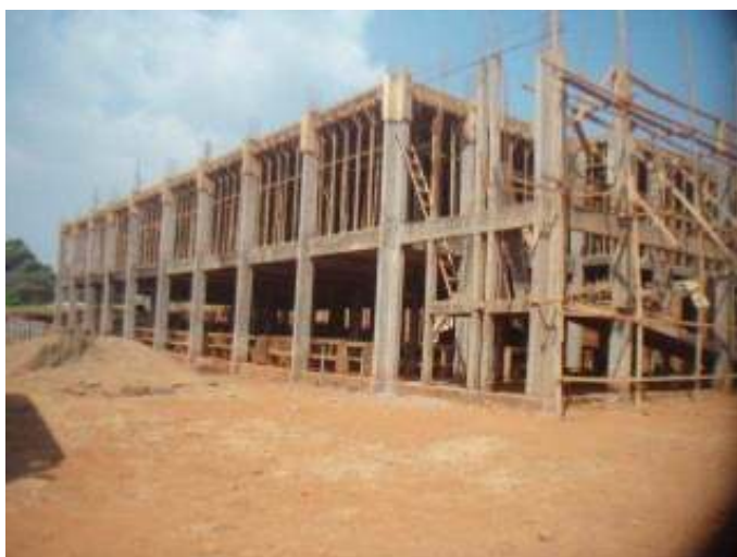
PTSFHP Building Under Construction
