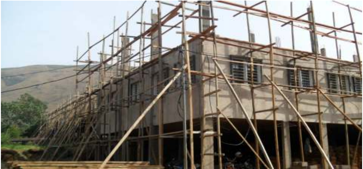
MBH NEW OPD UNDER CONSTRUCTION – SIDE VIEW
