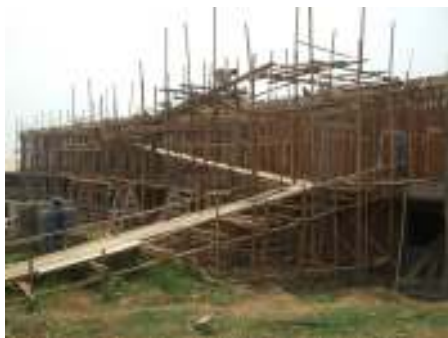
BHM Maternity Block Under Construction
